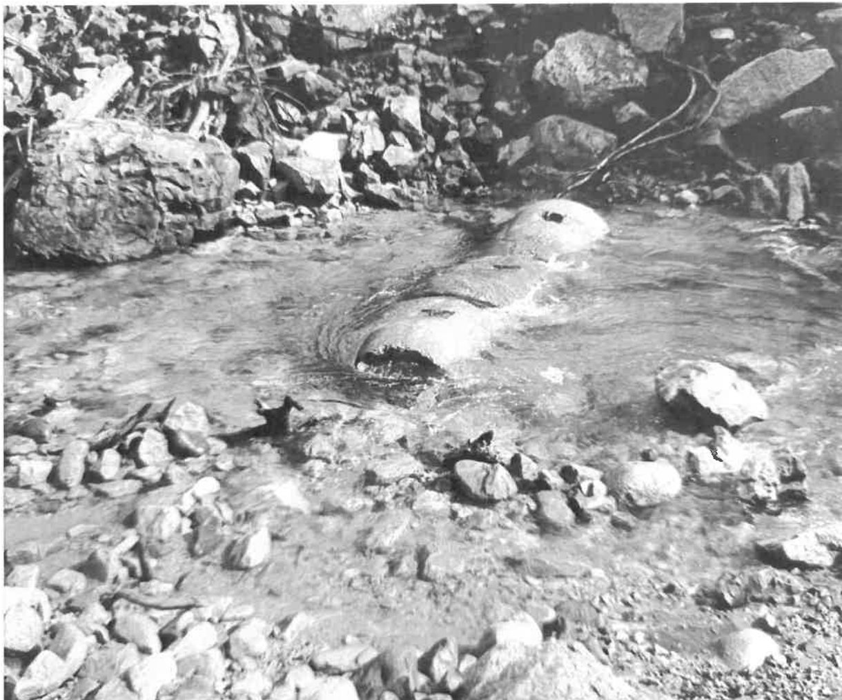
Concrete river weights were placed above Trans Mountain pipeline exposed in the Coquihalla River after flooding in 1995.
